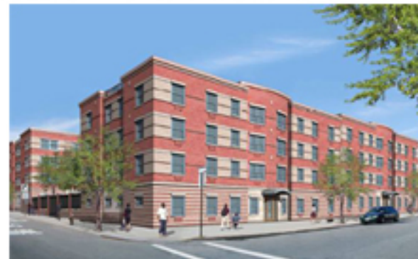
GREEN ROOMS: Habitat for Humanity is working on 41 LEED-certified condos in Brooklyn.
