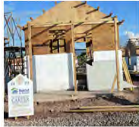
A new Habitat home under construction, to be finished in January.
